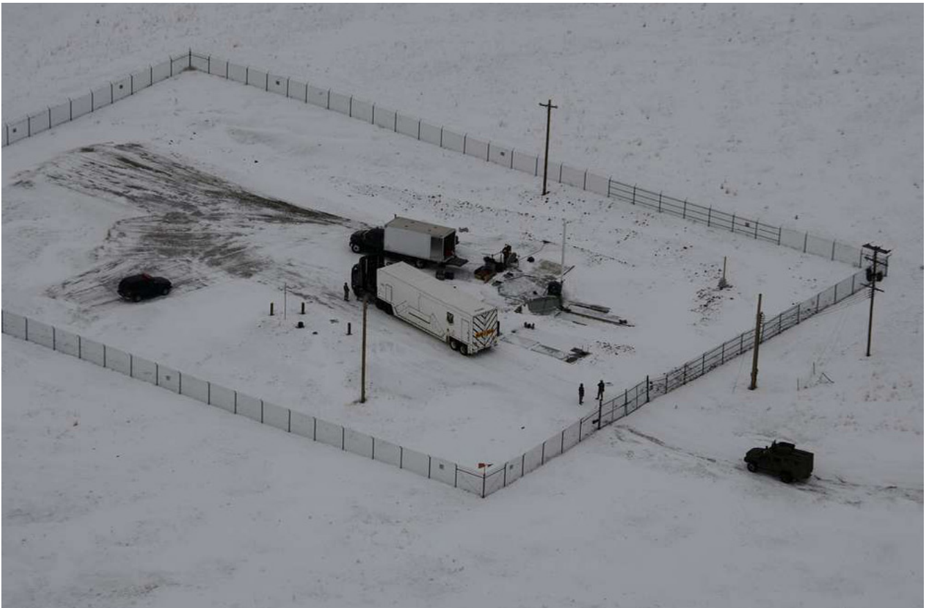
U.S. Air Force 341st Missile Maintenance Squadron transports a new re-entry system to be installed at an Intercontinental Ballistic Missile launch facility near Malmstrom Air Force Base, Mont. Public domain.
